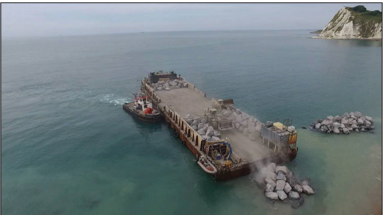
Figure 7b: Charlie Rock discharging rock armour
