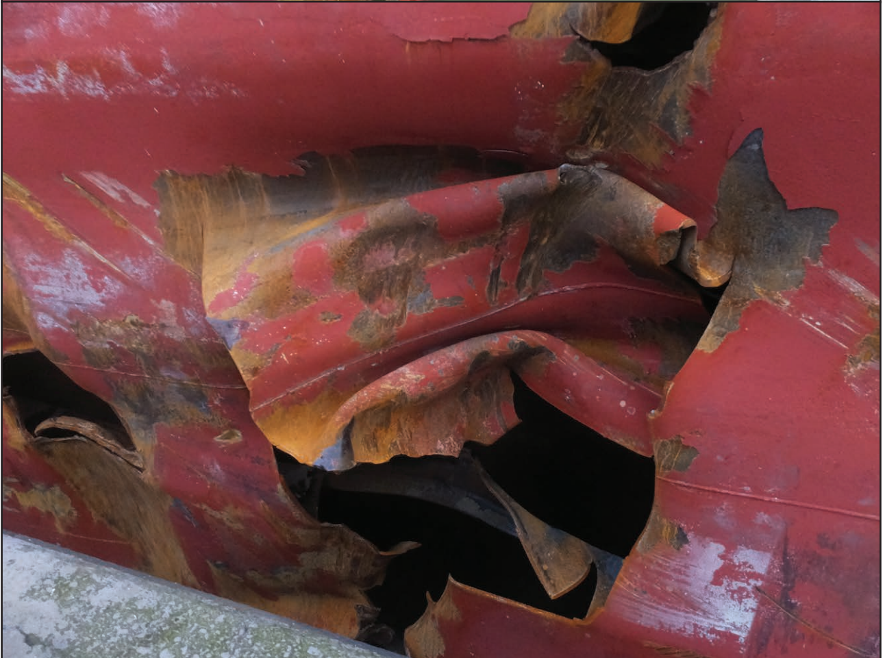
Figure 3a and 3b: Damage to Saga Sky's starboard side
